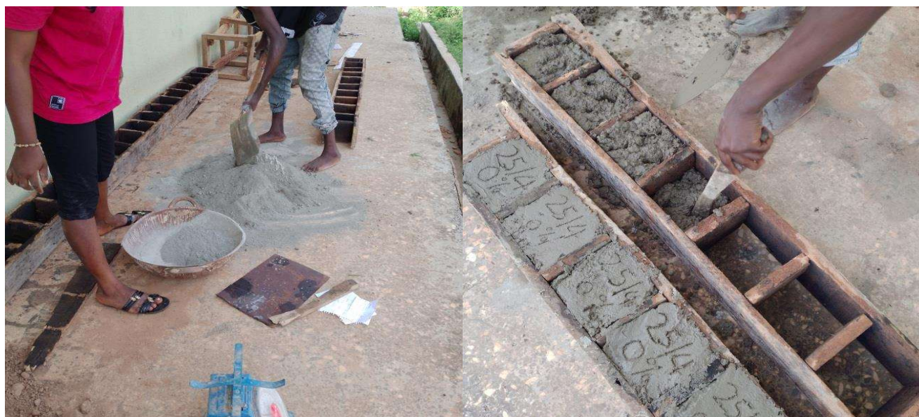
(a) Mixing of the Concrete
